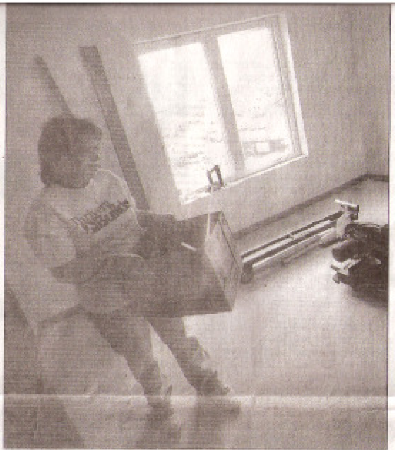
Schalon Schleicher of West Bend stands in a bedroom in one of the units at the Miller Street Habitat for Humanity site in West Bend.
